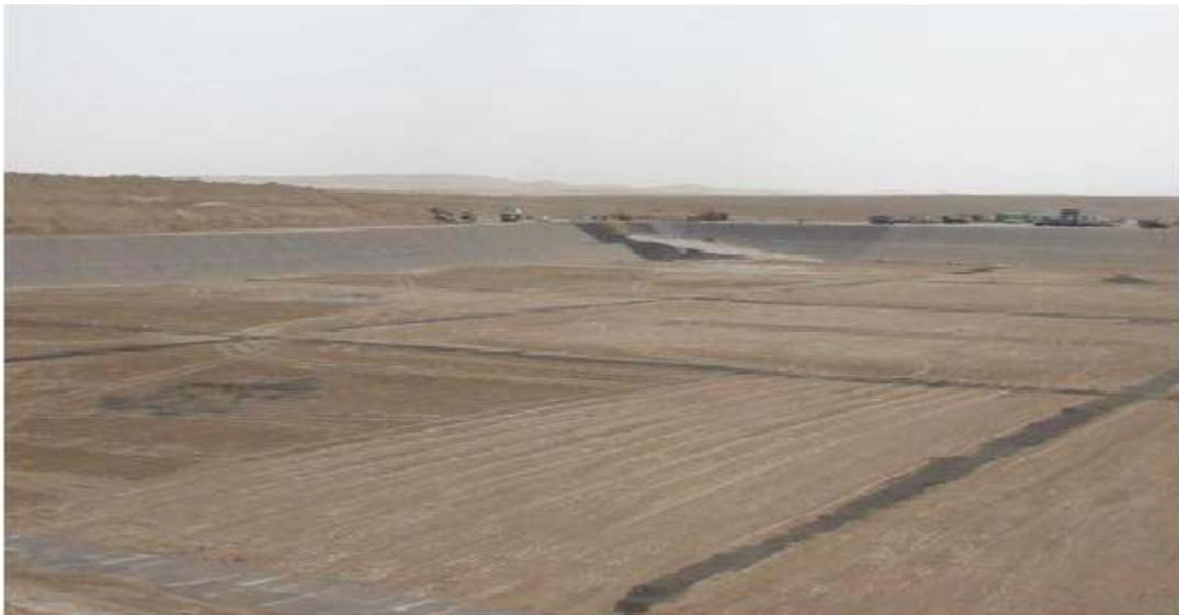
Figure (9): Final stage of lining at the cell of Ghabawi landfill
