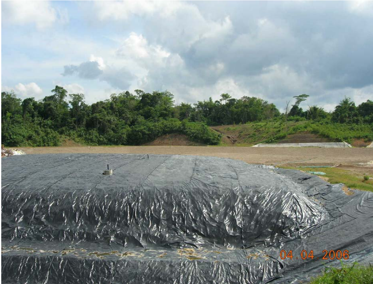
Figure 3. Surface cover with HDPE liner
