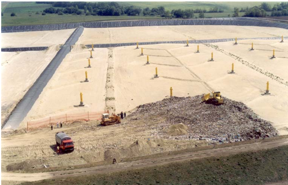
Figure 4: Aerial photo taken during the first placement of waste in 2000 with the gas wells. The gas wells variant implemented in 2000 with a continuous gas extraction from below, taking a short-term effect, turned out to be very susceptible to the condensate level in the landfill body on the occasion of gas extraction tests in 2006.
