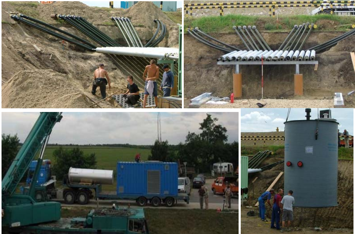
Figure 8: Construction phase in July and August 2006
