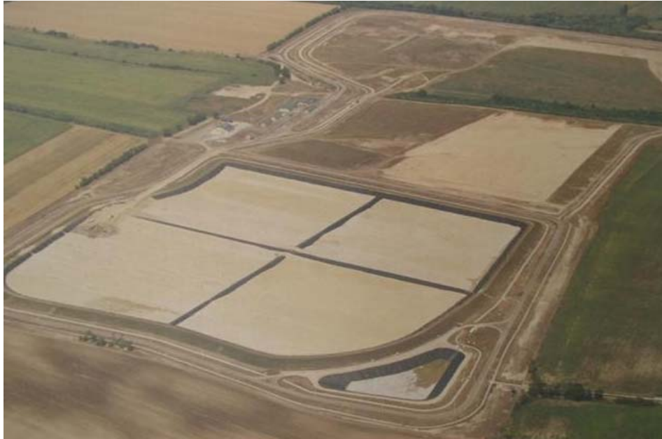
Figure 3: Aerial photo, taken during the construction of the landfill in 2000
