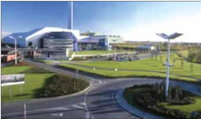
Fig. 4: Brescia WTE plant. The plant produces 650 kWh electricity per ton MSW combusted. [Themelis, 2003]
