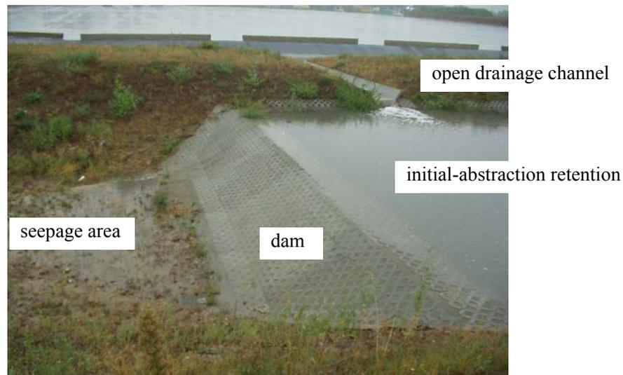
**Figure 5:** Open drainage channel (in the background), seepage treatment (in the foreground)
