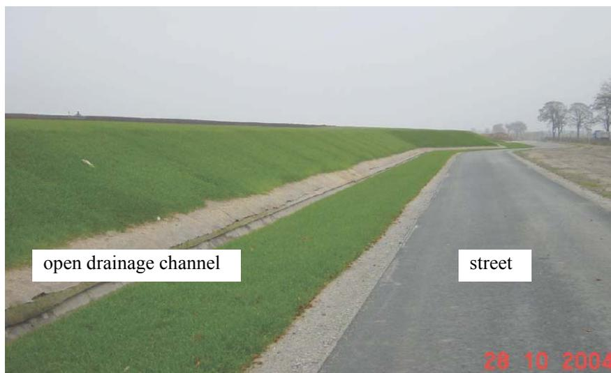
**Figure 6:** Landfill border street with open drainage channel
