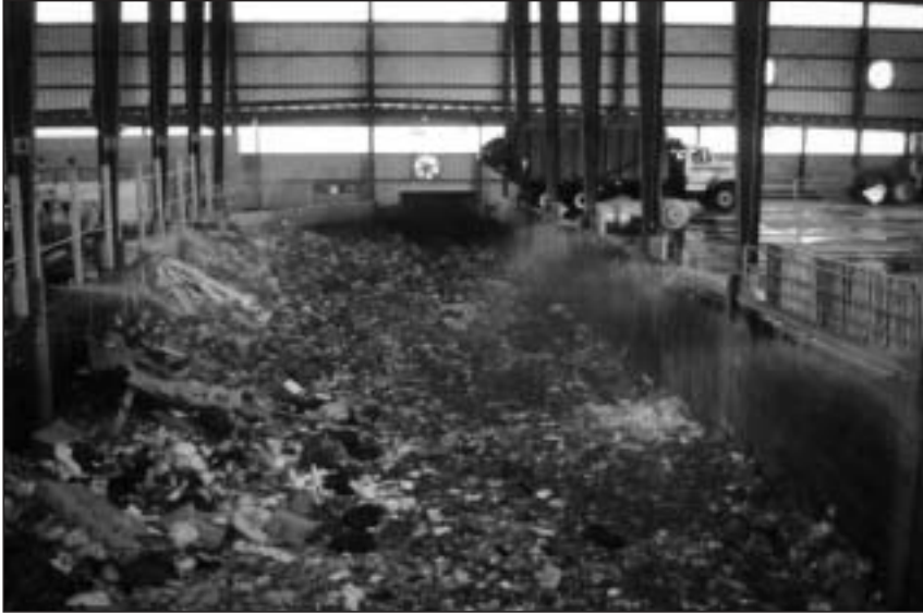
Surge pit separating public and commercial vehicles. Water sprays along the walls of the pit are used to suppress dust.
