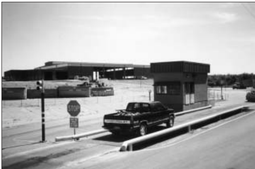
A transfer station scale house.
