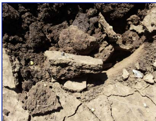
Poor soil structure
