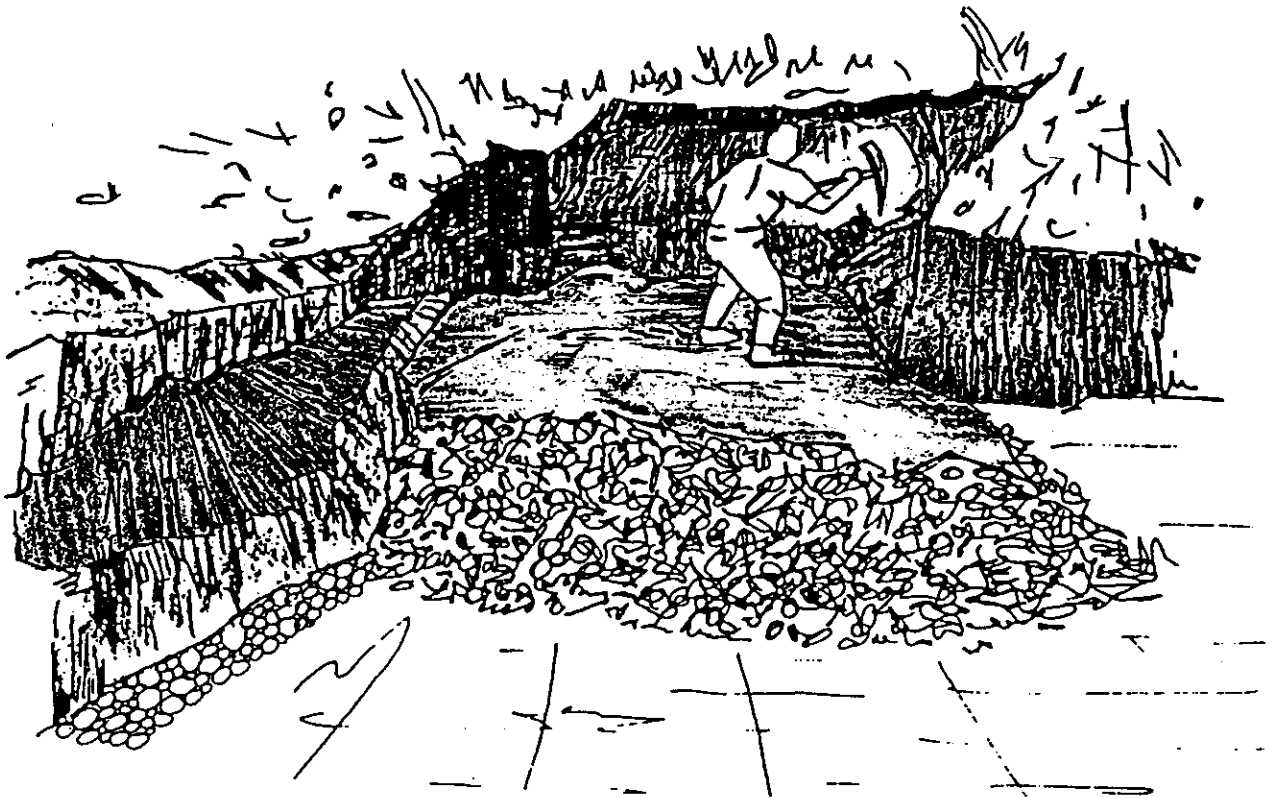
FIGURE A.4 EXTRACTION OF SOIL FOR COVER
