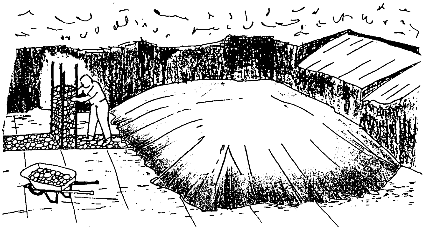
FIGURE A.7 CONSTRUCTION OF A GAS VENTING SYSTEM
